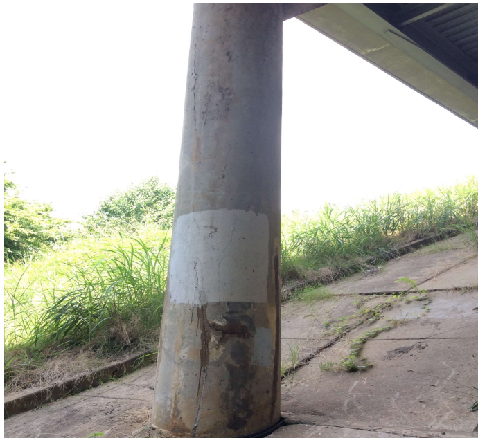
PHOTO 1 Description Bent 3, Column1 patched area
