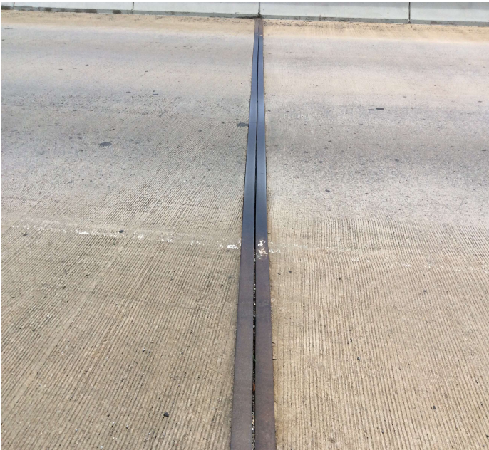
PHOTO 1 Description Expansion joint seal over Bent 2.
