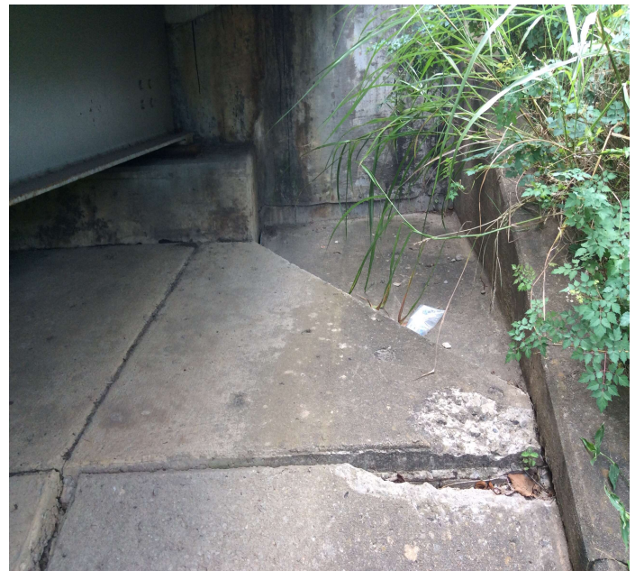
PHOTO 2 Description Concrete riprap adjacent to Bent 1.
