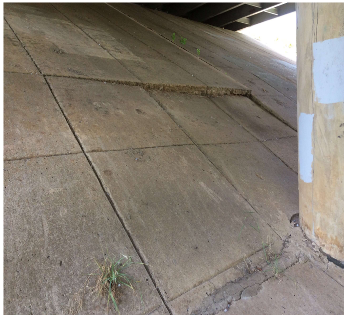
PHOTO 1 Description Concrete riprap under Span 3.
